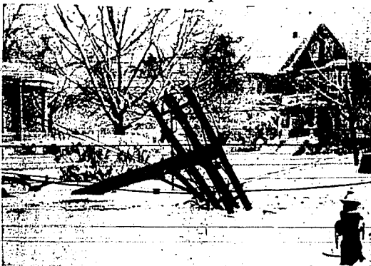
This scene at Somerville, Mass., is typical in many New England towns as recent heavy snows caused collapse of hundreds of utility poles, causing power failure and the danger of live wires in the streets.—(NEA telephoto)
