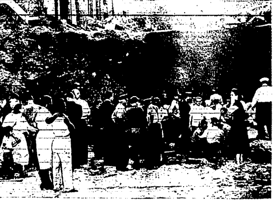
Here is a general view of the scene at the cave-in at the side of cut for the Brooklyn-Queens expressway in New York where six youngsters lost their lives when tons of earth fell on them in a cave in which they were playing. Anxious relatives and friends watch as rescue workers, right, try in vain to revive the children. (AP Wirephoto)
