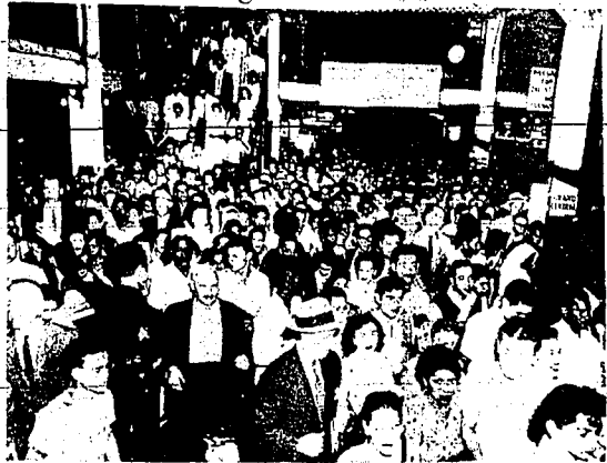
Thousands of people jam the Grand Central subway station in New York in one of the worst commuter jams in the city's history. They were forced to use alternate routes when subway stations were flooded by the water used in fighting the 25-hour fire at the Wanamaker department store building. (AP photo)
