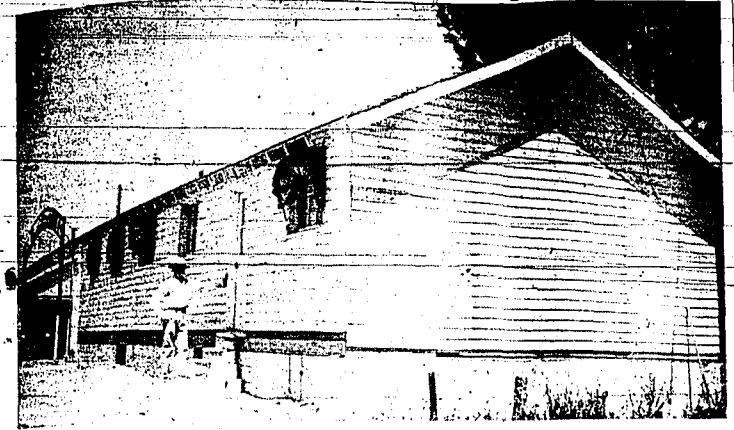
The Secretary Tom Parks stands beside the partially completed fair office building at the Twin Falls fairgrounds in Filner. The building was removed from its foundation while a basement was dug and then replaced. The next step, expected to start sometime this week or next, will be to cover the building and the entrance to the grounds with a rock or brick veneer. (Staff photo—enr.)
