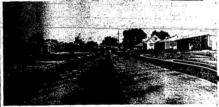
Eleventh avenue east between Morningstar drive and Highview lane is one portion of the seven miles of Twin Falls streets affected by this year's $100,000 street improvement program. The street is shown here ready for paving. (Staff photo-engraving)
