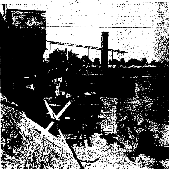
The new city asphalt mixing plant, located south and east of Five Points east, is capable of turning out 750 tons of blacktop a day for the $100,000 street improvement program in Twin Falls. The mixer puts out a five-foot-wide, five-foot-deep asphalt every four minutes. (Staff photo-engraving)
