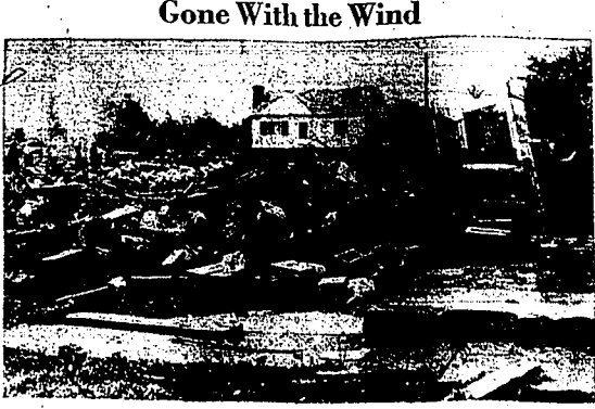
The home of John Reapsummer is a mass of rubble after it was leveled by a tornado which struck Girard, O. Living in the basement for six years, the house was being completed. Reapsummer, his wife and three children were not injured. They were to move upstairs in a week. (NEA telephoto)
