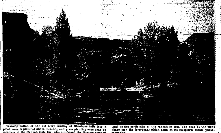
Transformation of the old ferry landing at Shoshone falls into a picnic area is pictured above. Leveling and grass planting were done by members of the Canyon club, Inc., who purchased the 90-acre area of land on the north side of the canyon in 1952. The dock at the right floats over the ferryboat, which sank at its mooring. (Staff photo-engraving)
