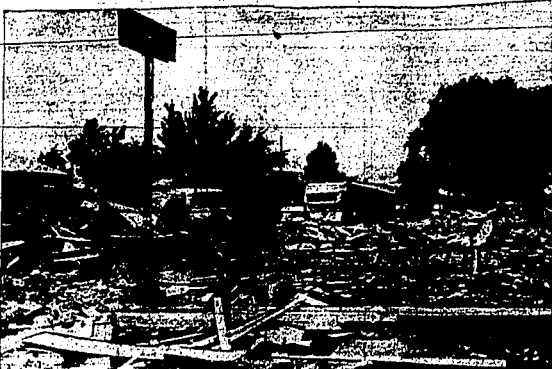
This rubble is all that remains of the Earl's cafe in Monticello, Utah, after an explosion ripped the brick and cinder block building apart during the busy dinner hour. At least 15 were killed and 28 injured in the blast, believed caused by leaking gas, which brought shock and sorrow to the milling community in the southeastern part of the state. The sign, mounted on a pole, is all that remained standing. (AP Wirephoto)
