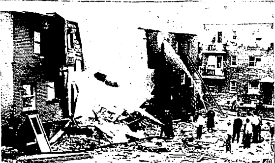
This is all that is left of an apartment building at Montreal, Que., after it was torn apart by a terrific explosion when a gas main broke. The building was turned into a raging inferno in which eight persons were killed and at least 15 others were injured. (AP wirephoto)
