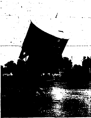
This Union Pacific railroad water tank, in use in Durley since 1909, was toppled Wednesday since it no longer is needed. The tank, with a capacity of 50,000 gallons of water, was used by many steam locomotives before the advent of diesel engines. To bring the tank down, railroad employees simply jacked its legs from under it. This picture was snapped as the tank began to fall. (Photo by Bob Lynch—staff engraving.)
