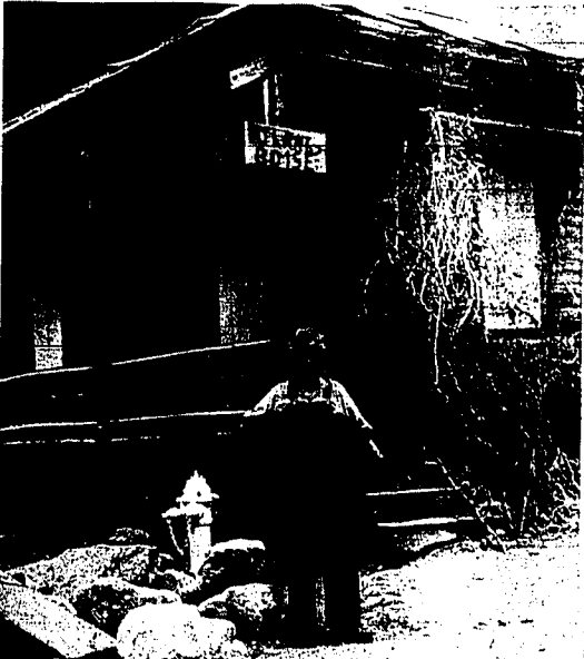
Charles Sprittles, who says he's the mayor of Rocky Bar, stands by the community's "busted" mine. That beside him, believe it or not, is a fire hydrant. The hydrants were installed in the 1890's, costing quite a sum for the time. Residents then felt secure against fire but on the day after the installation was completed the top was knocked over and the fire almost burned the town down because the hydrants didn't work. Sprittles runs the general store and, in addition to merchandise, will repair his customers with stars of the past. (Staff photo-enlarging)
