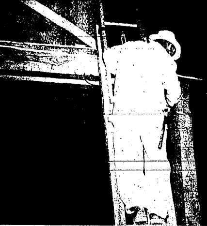
C. H. Vandier, Jerome, an employe of Reynolds and Walker Construction company, examines the split discovered Monday morning in two overhead beams in the northwest corner of the Twin Falls High school gymnasium. The beams were replaced by a new beam of the same size and shape. The beams were replaced by a new beam of the same size and shape.
