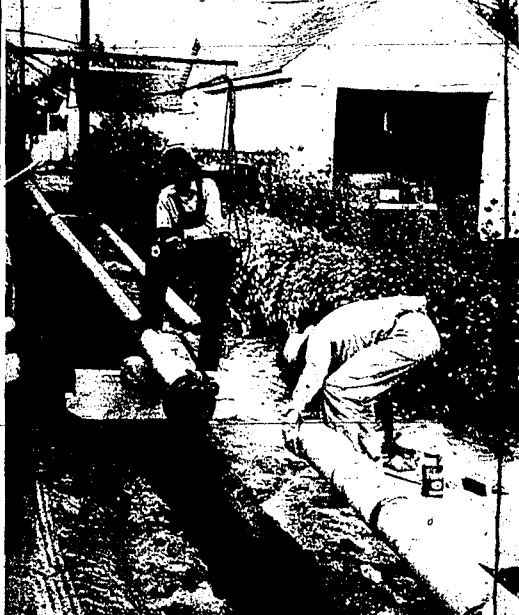
Laying of natural gas network distribution system began in Twin Falls Monday morning in the alley between Third avenue and Fourth avenue east. Jack Norris, area engineer for Pan Service and Management corporation, said either crew started in different locations Tuesday. A workman prepares to splice a length of pipe. The system will have a minimum cover of 36 inches. (Staff photo-enlarging)
