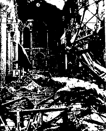
Only skeleton-like walls remain after a two-million dollar fire destroyed the Episcopal church, a Roman Catholic church in Cambridge, Mass.
