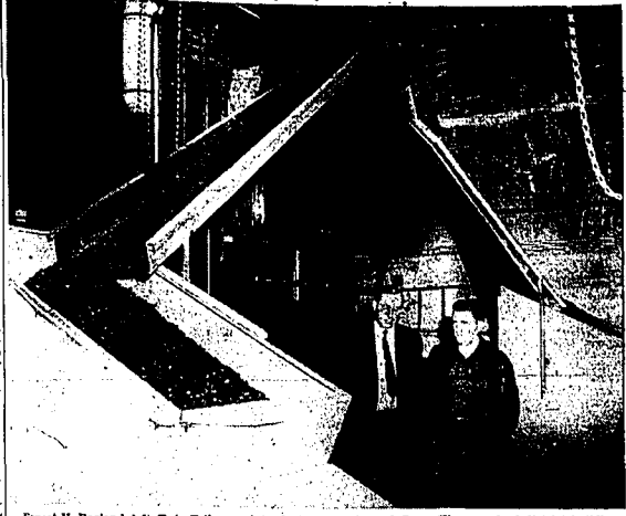
Ernest H. Ragland, left, Twin Falls superintendent of schools, and Owen Kinney, school district buildings and grounds superintendent, are shown with the recently-installed double boiler heating system at the junior high school...
