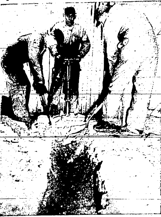
Digging for a broken water pipe when the ground is frozen is almost like digging through solid concrete as evidenced by Glenn Brown, running the jackhammer, Gene Harr, kneeling, and Leroy Harr, using the shovel. Often dynamite is used by city water department men to break up hard ground, according to J. H. Latimore, Twin Falls city manager. (Staff photo-contrast)
