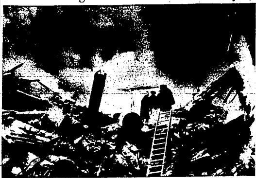
Fire chiefs hold conference amid the smoldering ruins of a twin and paper factory which collapsed at the height of a five-alarm blaze in New York. Two firemen were known dead and four others were trapped and presumed dead in the wreckage of the six-story building. (NEA telephoto)
