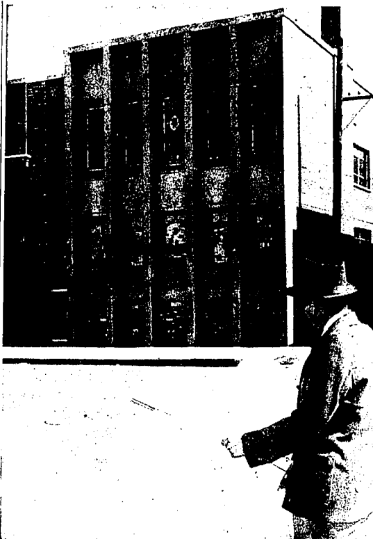
The finished product looks like this built from the plans of Harold E. Gerber. He relates that it takes at least two years of college, three years of apprenticeship and successful completion of a four-year state exam to be licensed as an architect. (Staff photo-engraving)
