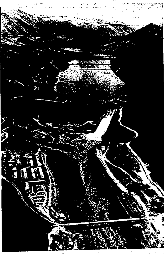
The reservoir behind Brownlee dam is filling preparatory to start of generating 200,000 kilowatts of electricity. Power plant is located at left side of dam. On the right, or side, water pours through lower gate of spillway. (Idaho Power company photo—staff engraving)
