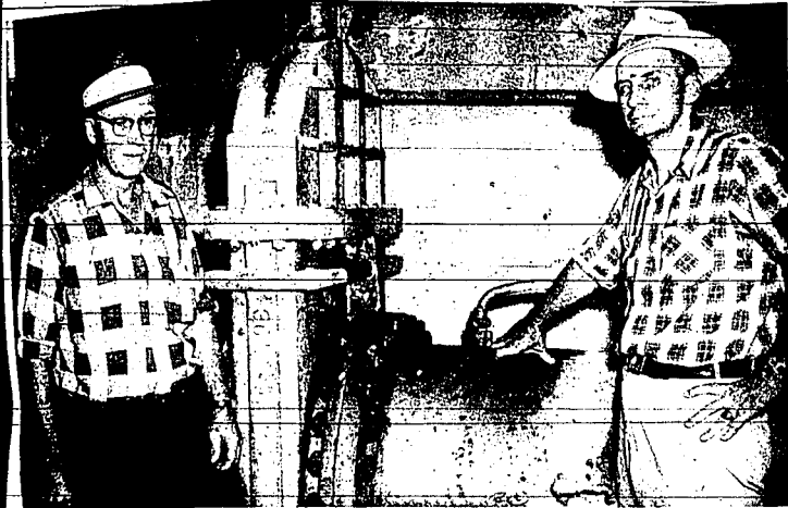
Kenneth R. Leazer, filter plant foreman for 18 years, and Wayne E. Koenig, a plant operator, show the relative size of the water main leading into the Twin Falls filter plant south of the city. The 42-inch inside pipe has a large valve to control the amount that enters during repairs or cleaner. The plant produced 1,791,284,000 gallons of water last year, all of it flowing through this pipe. During the summer months the Willow Lane well helps alleviate water shortages. (Staff photo-encouraging)
