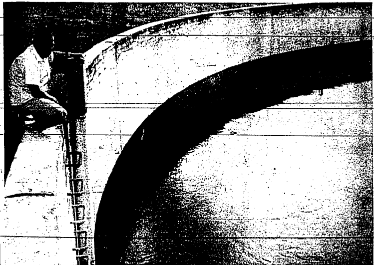
City manager Joseph H. Lattimore checks water depths in reservoir south of Twin Falls. He had read upon a metal line containing gauge which records the amount of water. The steel ladder which goes to the bottom of the 20-foot reservoir has 20 steps at one-foot intervals. The water in the 20-foot diameter concrete structure is crystal-clear. The bottom is always visible. Ten feet of the reservoir is above ground, and 10 feet is below the surface. The reservoir was built in 1923 and has a capacity of five million gallons. On week-ends the reservoir is usually full, but by late Monday morning, the water has dropped several feet. It remains below capacity when more water is being used than is produced in the filter plant, a common situation in summer. (Staff photo-engraving)
