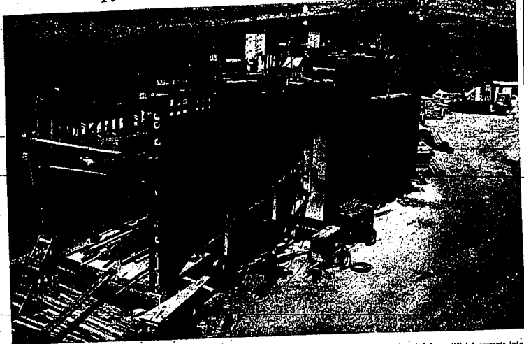
Some 600 miles from the sea as the gull flies, this "shipyard" at Brownlee dam is busily building three of the oddest craft ever to take to water. They are the ingenious floating "skimmers" or traps, that literally will scoop salmon and steelhead fingerlings from the water as part of the costly downstream-migrant fish facilities Idaho Power is installing in Brownlee's reservoir. Fabricated of steel, each company is installing in Brownlee's reservoir. Fabricated of steel, each company is installing in Brownlee's reservoir. Fabricated of steel, each company is installing in Brownlee's reservoir.
