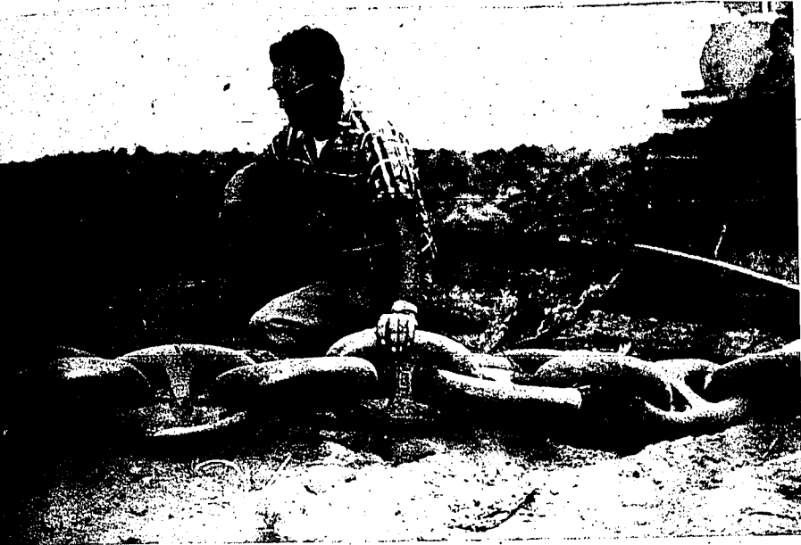
Walter C. Higgins, technician with the Twin Falls soil conservation service office, stands by the former navy anchor chain which the Twin Falls soil conservation district uses on the sagebrush desert southwest of Hollister. Each of the 80 links in the heavy chain weighs 65 pounds, including the steel H-beam to which the chain is connected at each end, the massive equipment weighs about four tons. Purpose of the equipment is to break down the sagebrush or pull it up. After that, the brush dies and valuable soil nutrients and moisture are saved for Siberian wheatgrass which is planted on the range land. The drag makes an 18-foot wide, clear about five acres per hour. (Staff photo-engraving)
