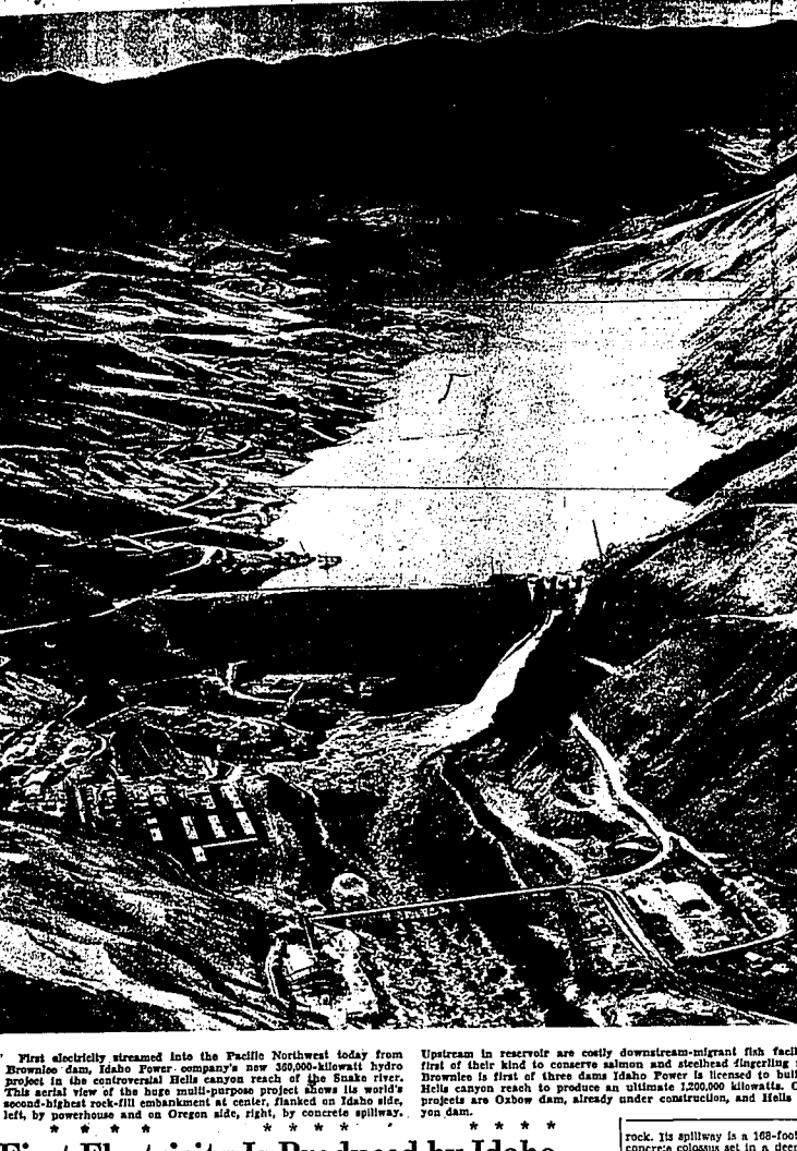
First electricity streamed into the Pacific Northwest today from Brownlee dam, Idaho Power company's new 350,000-kilowatt hydro project in the controversial Hells canyon reach of the Snake river. This aerial view of the huge multi-purpose project shows its world's second-highest rock-fill embankment at center, flanked on Idaho side, left, by powerhouse and on Oregon side, right, by concrete spillway.
