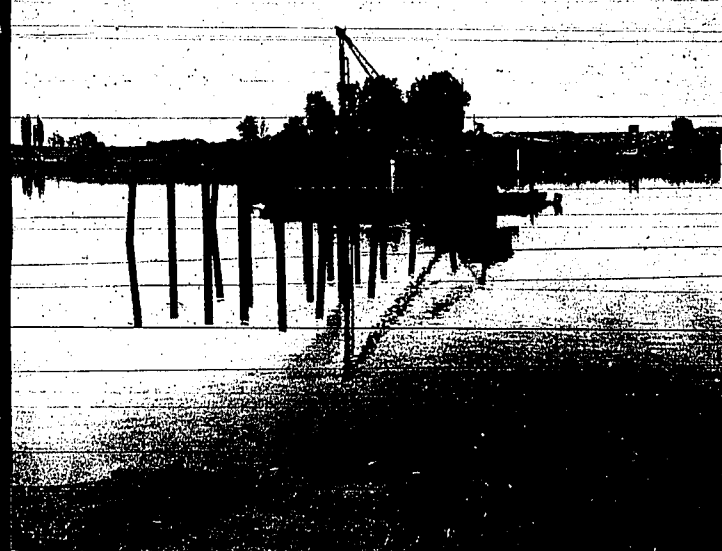
Here's start of 372 piles which will support new parallel bridge across Snake river north of Declo and south of Highway 30N-highway junction. At the average of eight piles per day, it is expected that piles will be driven in two and one-half months. They are 22 to 40 feet long, with 15 to 18 feet planted beneath the river bottom. After all are driven, they will be trimmed to elevation, filled with concrete and capped. Operations were begun from the middle of the river. (Staff photo-enslaving)
