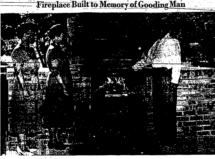
Workmen building the fireplace and holder of public utility who died May 13. Feels in front of memorial are a son and two daughters. Floyd Thornton, route 1, Gooding; Mrs. Jack Craig, Glenn Ferry; and Mrs. Madeline Stokes, Buhl. The structure was used for the first time last Sunday. (Staff engraving)
