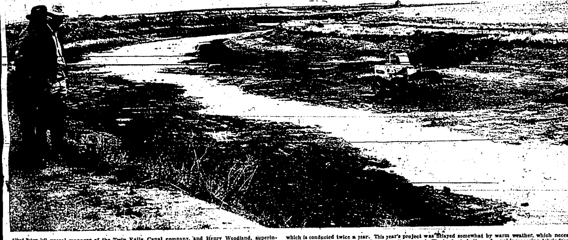
Alfred Peters, left, general manager of the Twin Falls Canal company, and Henry Woodland, superintendent of construction, discuss canal repair problems during the time last week when the canal system was drained. Twice each year, the entire canal system is drained for inspection, maintenance work, repairs and debris are removed. Last week, water was turned out of the canal system for four days for work which is conducted twice a year. This year's project was delayed somewhat by warm weather, which necessitated use of water for bed fields longer than usual. The leader in bottom of canal is removing debris from the channel. Soil and rock removed from the channel are used to build up banks along canals. (Staff photo-enslaving)
