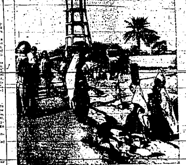
Water tower under construction in old city area.
