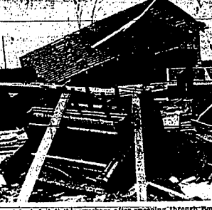
Powerful winds left this wreckage after sweeping through Bowler in central Oklahoma this week. Pictured here is the remains of a Methodist church with an unroofed piano in the debris.
