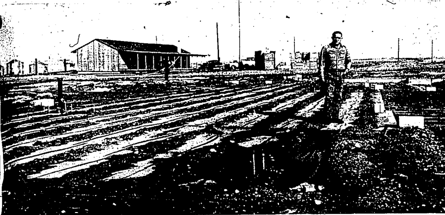
The Rev. James H. Crowe, superintendent of the Idaho Ranch for Youth, stands on the foundation of the ranch home unit now under construction. About $15,000 in cash will be needed to buy materials for the interior partitions, windows and roof. There is sufficient material for the walls, but construction can't be continued until all materials are on hand. In the background is the main ranch building, the only living quarters presently available on the ranch. (Staff photo-engraving)
