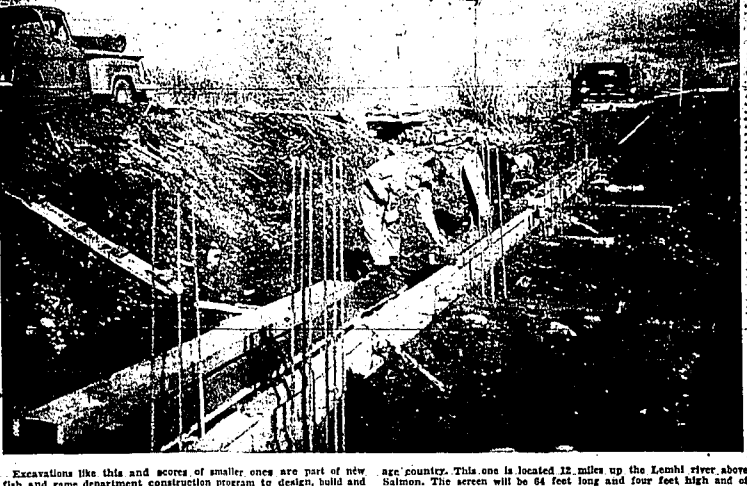
Excavations like this and scores of smaller ones are part of new fish and game department construction program to design, build and install some 250 automatic fish screens to prevent fingerling salmon, trout and other species from going down irrigation ditches to ultimate destruction. Although 10 screens already are operating on the Lemhi river, this is a five-to-seven-year program for the Salmon river drainage
