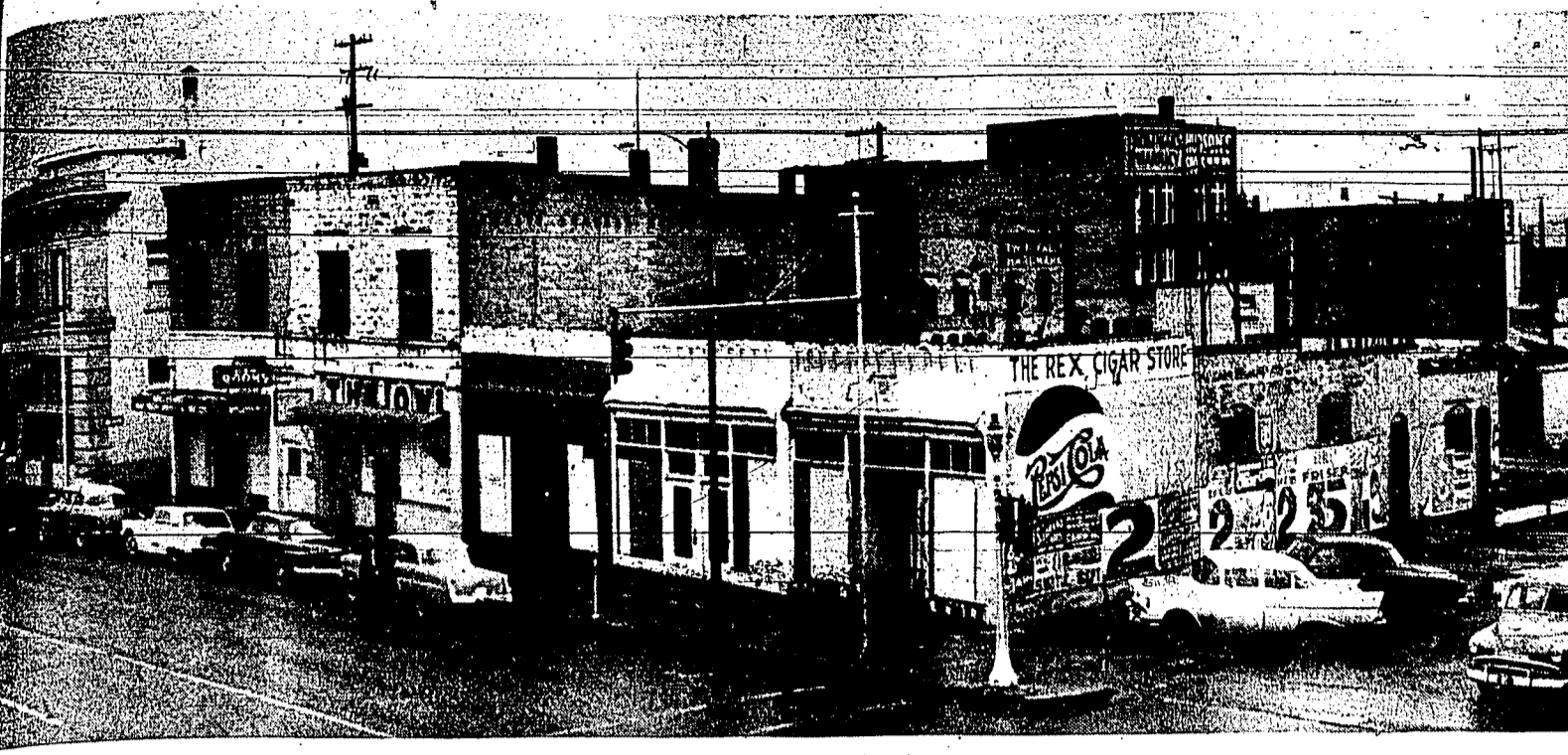
Within a month, razing operations will begin on this group of pioneer Twin Falls buildings on Shoshone street south. The entire half block of buildings will be leveled for roughly the same purpose since they were built. Weather permitting, by early June the Twin Falls Bank and Trust company will complete a drive-in branch and a new parking lot on the property between the bank and Second avenue south. Harry Eaton, president of the bank, says contracts will be let in the near future and razing operations on the 125-by-150-foot lot will begin within 30 days. Leveling of the old buildings marks the end of an era for some of the oldest buildings in Twin Falls. Records at the Boone Land title company show construction of
