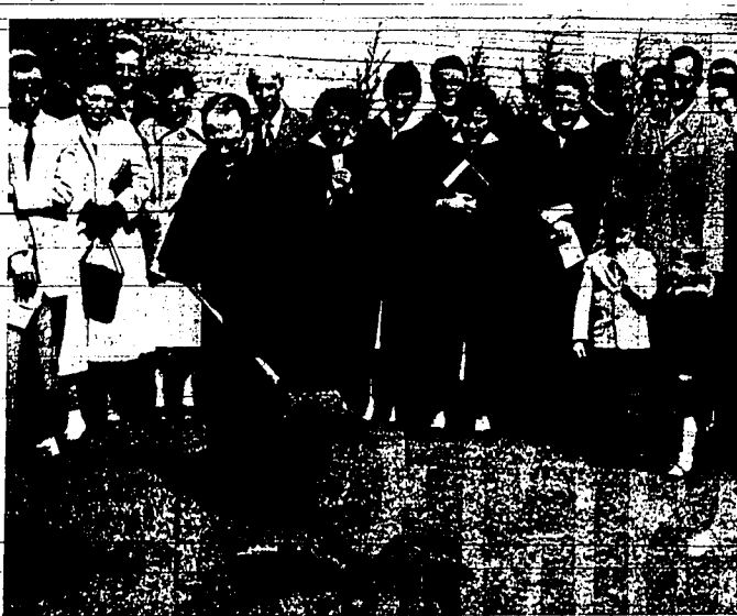
The Rev. Richard H. N. Yost, pastor of the First Methodist church at Twin Falls, turns the first spade of dirt on the site of the new $25,000 educational unit to be constructed by the Barley church. Grouped behind the pastor are, from left, Dr. D. V. Holcomb, member of the finance committee; Mark Moorman, church lay leader; Edgar Moorman, chairman of the board of trustees, and Glenn Berryman, charter member of the church and chairman of the finance committee. All of whom participated in the ground breaking ceremony Sunday after church services. Actual work started on Monday, March 16.
