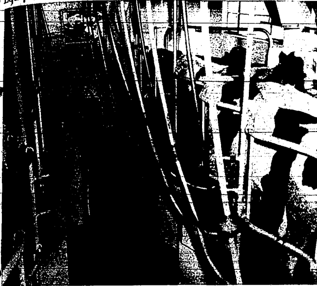
J. C. Williams, Twin Falls, works in the pit of his ultra-modern milking parlor. The cows on the right are being milked and the milk is transported through overhead flyer pipes and conveyed into a 1,000-gallon bulk milk tank in the next room. While
