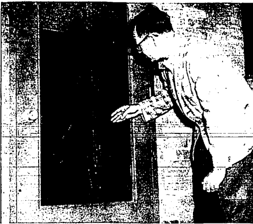
Twin Falls high school Principal V. L. LeFebvre examines door on school's north side that was smashed by vandals early Tuesday to gain entrance to the building. From a small fire safe in the home economics room and the school reception area, a total of $31.25 was taken. A soft drink machine in the teachers lounge was pried open and coins taken from the collection box. School supplies were strewn on the floor in two or three of the school's rooms. City police took fingerprints from the door of the fire safe. (Staff photo-entwring)
