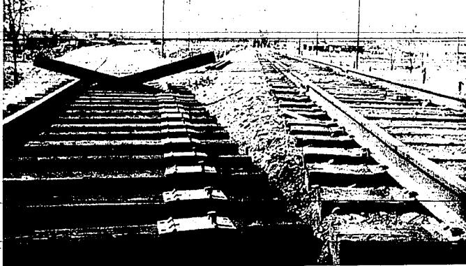
Union Pacific Railroad company trains will be diverted onto the "shoofly" track branching to the left of the main track during construction of the $108,500 underpass on Eastland drive just south of U. S. highway 20. A railroad crew removed the main track Tuesday afternoon at the Eastland drive railroad underpass project just south of U. S. highway 20. In the background is the excavation already completed for the underpass project. A few yards south of the present track, a "shoofly" track has been constructed to allow trains to pass the project site. The underpass, costing $108,500, will be 25 feet wide, one-third of a mile long and provide for two lanes of traffic. Work must be completed sometime during July by Nielsen and Miller Construction company, prime contractors. (Staff photo-entourage)
