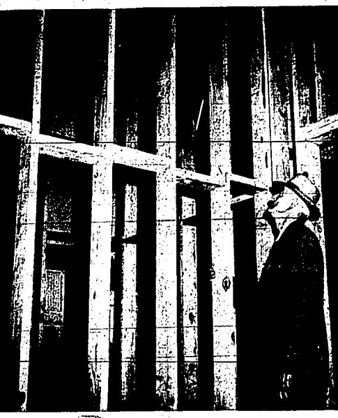
Frank Fonda, hired by county commissioners to supervise remodeling of the 48-year-old courthouse, inspects changes being made on the building's third floor. A partition is being erected in the present prosecuting attorney's office to provide space for the county law library and the prosecutor. Fonda expects work on the $4100 project will be finished next week. (Staff photo-courtesy)
