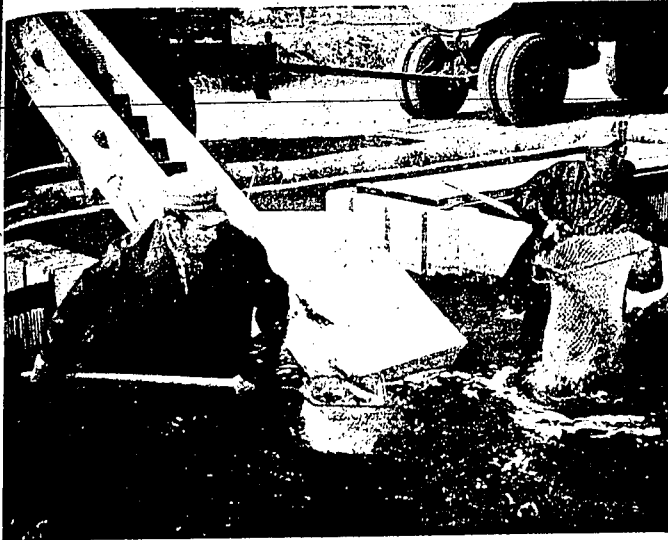
Two state fish hatchery helpers in the raceway at the foot of the automatic fish conveyor chain lift perhaps 20 pounds of trout with each net-lift and dump them into a water-filled hopper where the only way out is up. From there the fish and some water are lifted in the moving ladder to refrigerated compartments. (Idaho fish and game department photo—staff engraving)
