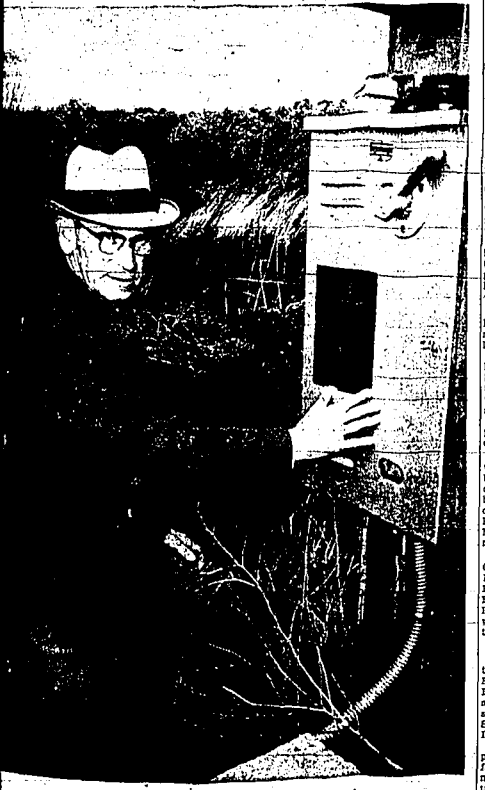
Caution. Power lines may be overhead. Look up before standing pipe on end. That's the warning by Harry Hamilton, Kimberly Idaho Power manager, on signs being placed on switch boxes near power lines. The long aluminum pipes used in sprinkler irrigation have been moved around much anymore and the chief danger involving derricks now results where farmers have located derricks near power lines. (Staff photo-entourage)
