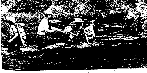
Wading with a telephone line, this photo illustrates the manner in which the middle fork of the Salmon river is forded across from the Sheepeater hot springs camp. A cable is stretched across the river and the Scouts and their supervisors lay the cable and cross the wide, hip-deep stream with the aid of the permanent staff, who stabilize the cable in the rushing current. These Scouts are just
