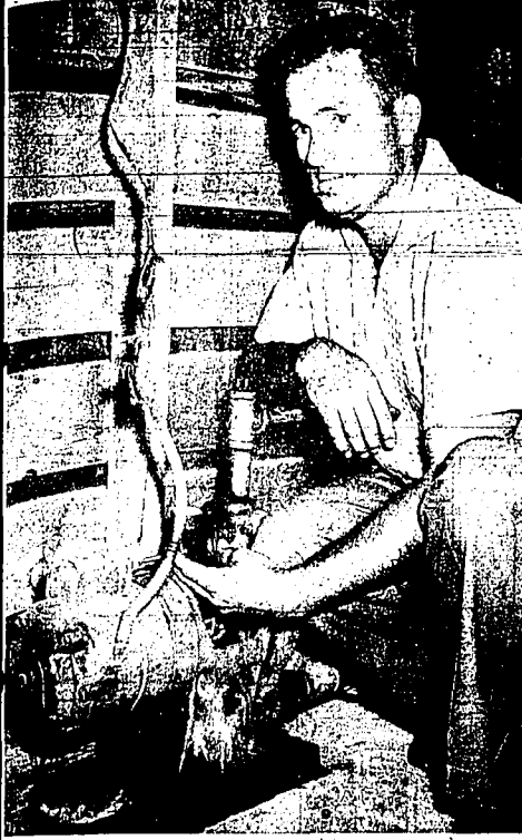
John H. Essary, 120 Lincoln street, oils the three-quarter horsepower pump that supplies most of the irrigation water for the Essary yard. The Essarys are some of the few lucky Twin Falls people who don't have to worry about alternate watering-days as ordered by the city commission. They have a flood-deep well with a six-inch casing that waters their 125-by-60-foot lot. Both Mr. and Mrs. Essary are that it's "very convenient" not to have to worry about alternate watering days. (Staff photo-graving)
