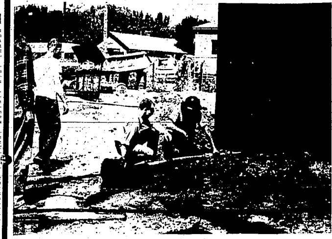
Jerome firemen check the connection of a gasoline hose that leaked and started a fire Friday morning at the Tins, Inc. warehouse in Jerome. A truck owned by Apache Tank Lines was filling the firm's tank when a spark from the engine used to pump gas into the tank ignited fumes. About 2,000 gallons of the tank's 1,200-gallon capacity were burned. When the picture was taken, flames had been extinguished and firemen were making final checks to be certain the fire wouldn't start up again. (Staff photo—enlarging)
