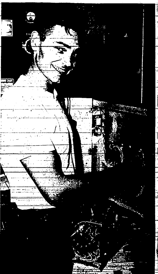
Gerald Smith, Los Angeles, crew chief with the federal aviation agency, works on new equipment installed at Joslin field as a navigational flight aid to pilots. It will give low-flying airplanes voice contact with the Burley FAA always traffic communication station. Previously, low-flying planes couldn't contact the station. Now they will be able to request weather information, file flight plans, and request emergency aid. (Staff photo-engraving)
