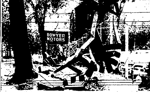
Gate force winds lashed away at the metropolitan area of Savannah, Ga., as Hurricane Gracie moved inland to the Charleston, S. C. area. This was a typical scene in Savannah as power was cut, communications down and traffic blocked. Many buildings have lost roofs and awnings as the 60-mile-an-hour winds continued to blow.
