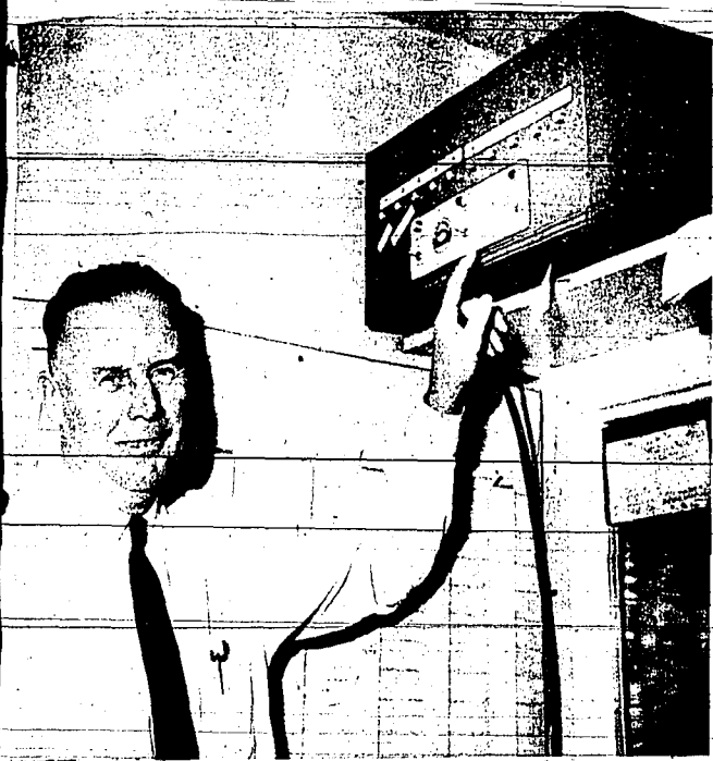
L. E. Bartlett, Twin Falls fire chief, points to a control box in the business that is part of a fire alarm system installed in several Twin Falls business houses in an attempt to lessen fire hazards. The control box is connected directly to an alarm system in the
