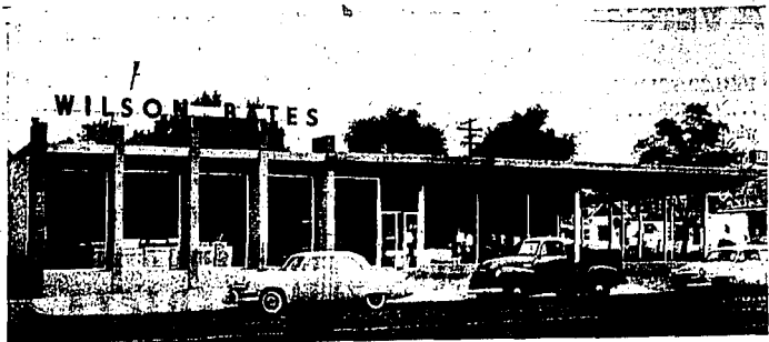
This is our Modern, New Home, located at the corner of Main Avenue and Seventh Street North. Brick and masonry construction. 100 feet by 100 feet in size, with laminated beam construction, acoustic tile ceiling, modernistic design and lighting throughout. Counter fronts, cabinets and cases of walnut and birch veneer. Wide-open windows affording daylight salesroom.
