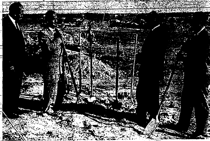
From left, President Ward Rawson, Jack Multhead, building superintendent; Bishop Vern L. Thomas and Howard Campbell, caretaker foreman, center on the project of building a $281,000 Blaine LDS stake center and chapel in Richfield. Footings were poured last week and Monday, volunteers will begin laying slender block siding. Neff Taylor, Salt Lake City, church architect, inspected the
