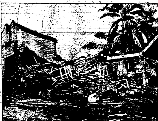
This is wreckage of one of numerous buildings caved in in Chihuahua, in the Jalisco state of Mexico, by the weak hurricane that struck along Mexico's Pacific coast in an area slightly larger than the state of New Jersey. The storm and the floods that followed took more than 1,000 lives, it is feared. (AP Wirephoto)
