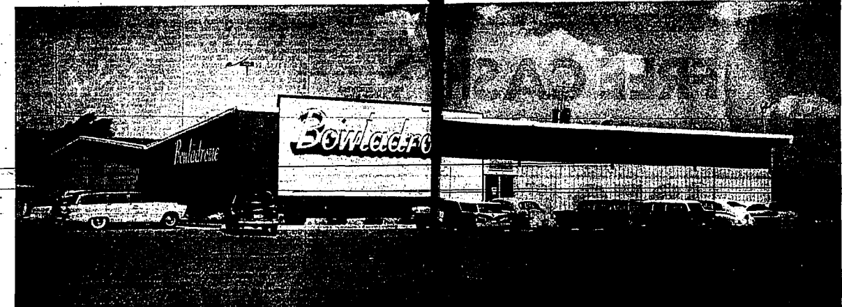
This is the exterior view of our modern, all steel, fireproof building with approach. The building's overall size is 120' by 145 feet with a clear open space of 100' by 120 feet single span for the alleys. It is located on 10th and DRIVE, east edge of Twin Falls, just south of Motor-Vu Theater.
