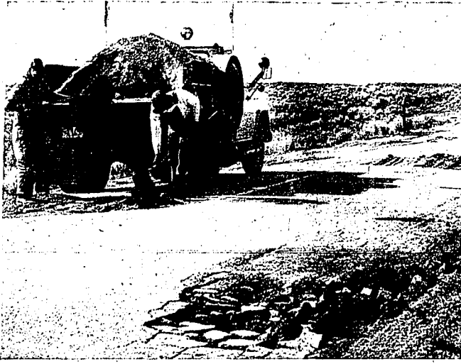
Idaho highway department maintenance men repair broken sections of U. S. highway 20 between Rupert and Traft river. After a warm and cold weather conditions with freezing and thawing have resulted in abnormally bad road surface breakup in many parts of the state this spring, Idaho department of highways plans to start repairs.
