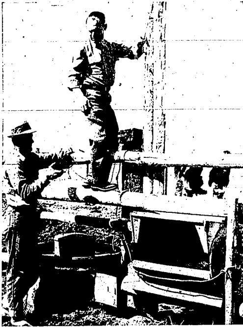
Checking wiring at this automatic waterer where two Holstein cows were killed because of faulty insulation are John Okelberry, left, and William Berry, Idaho Power agricultural representative. Okelberry passed the waterer that morning carrying a bucket of minerals for the trough on the right, and someone avoided contacting the "hot" water tank. (Staff photo- engraving)
