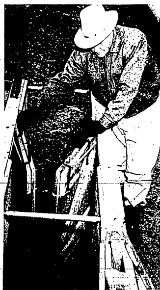
Warren Dalg, Twin Falls county agent, recommends highly this three-way portable sheep cutting gate. The portable unit was constructed on Ray Lincoln's winter headquarters south of Filer. It has a gate on each side and an opening at the front. It is about six feet long and two and one-half feet high, and can be transported on a pickup truck and used out on the range to sort lambs and ewes. (Staff photo-engraving)
